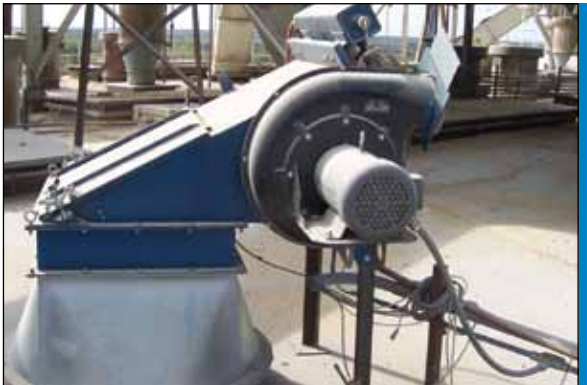
CPV-3 Grain silo bin vent (1200 cfm)
