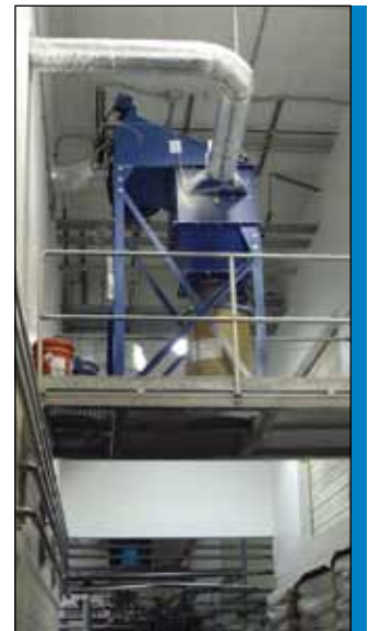
CPC-3 Powdered milk dust in cheese factory (1200 cfm)
