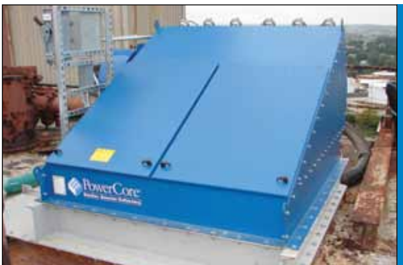
CPV-12 Cement silo bin vent conveyor (3700 cfm)
