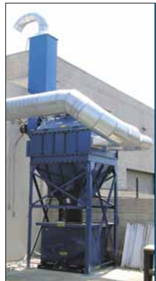
CPC-12 On wood dust at furniture manufacturer (7000 cfm)
